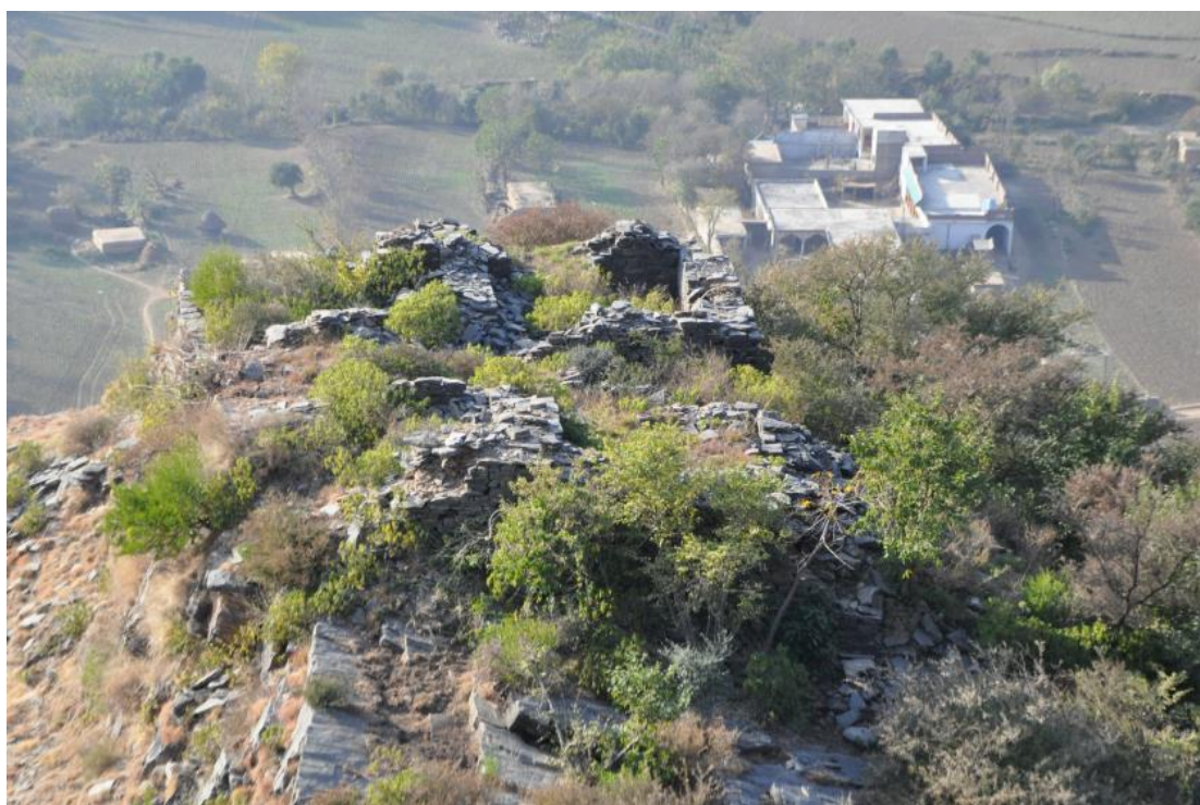
Fig. 13 – Shalbāṇḍai : Structural remains at the southern parts of Hamza Taṅgai Fort
