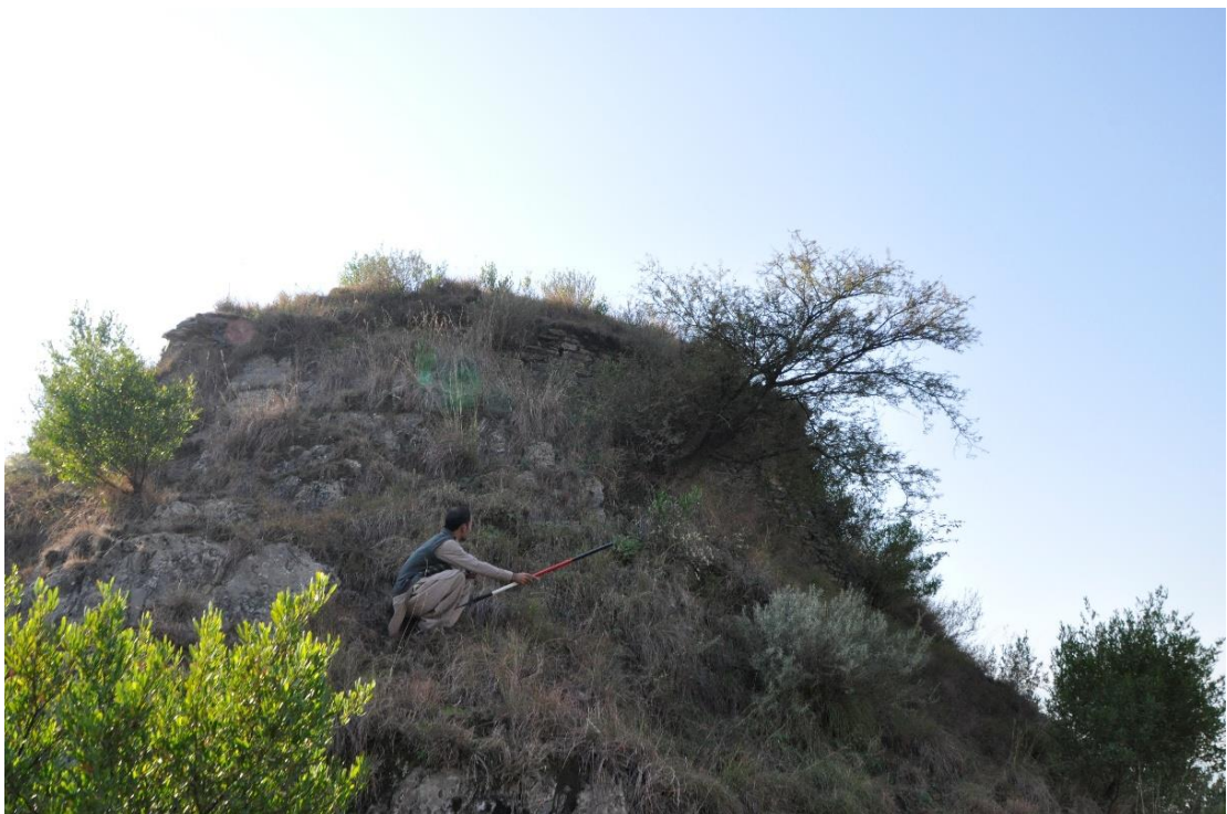
Fig. 25 - Shalbāṇḍai : Plinth of a breastwork or bastion at Lailā Site
