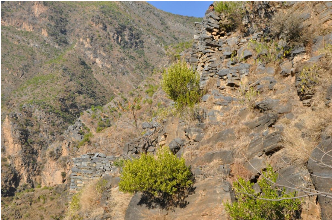
Fig. 27 - Shalbāṇḍai : View of the structural remains at Yakhdara Site
