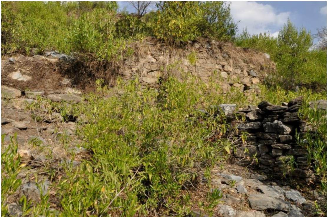
Fig. 20 - Shalbāṇḍai : Close view of the masonry work at Baḍais site
